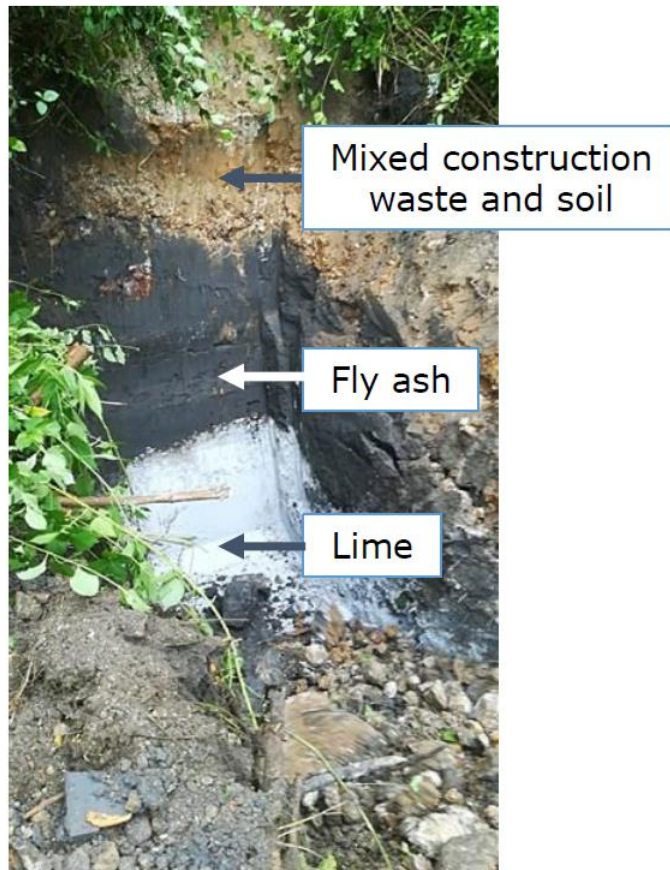
Figure 5-2 Trench performed at Onoz landfill showing inert waste, fly ash and lime (Credit Photo: Atrasol).
