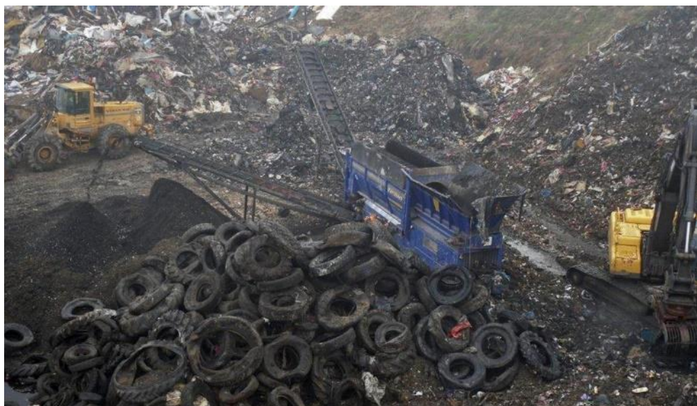
Figure 12-9 Landfill mining operations at Gerringe Landfill.
