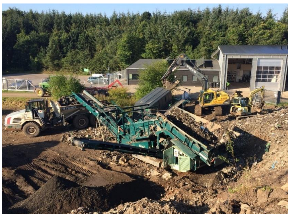
Figure 12-11 Landfill mining operations at Skårup Landfill.
