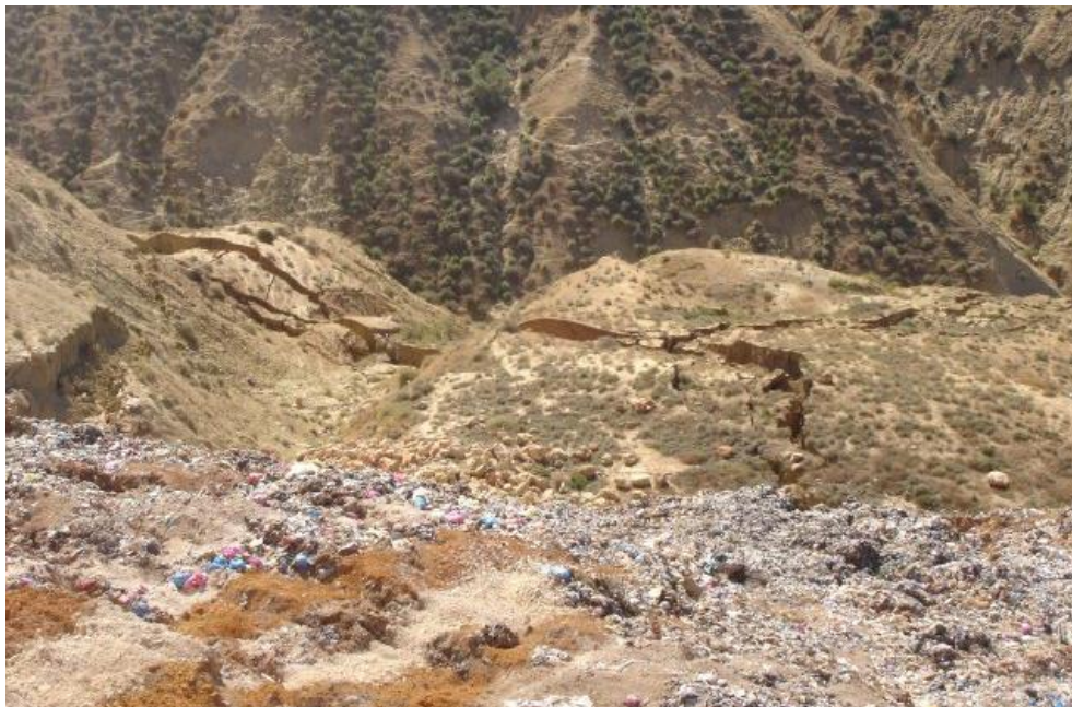
Figure 8-3 Destabilization of the bottom ground due to landfill slide (Credit photo: Atrasol).
