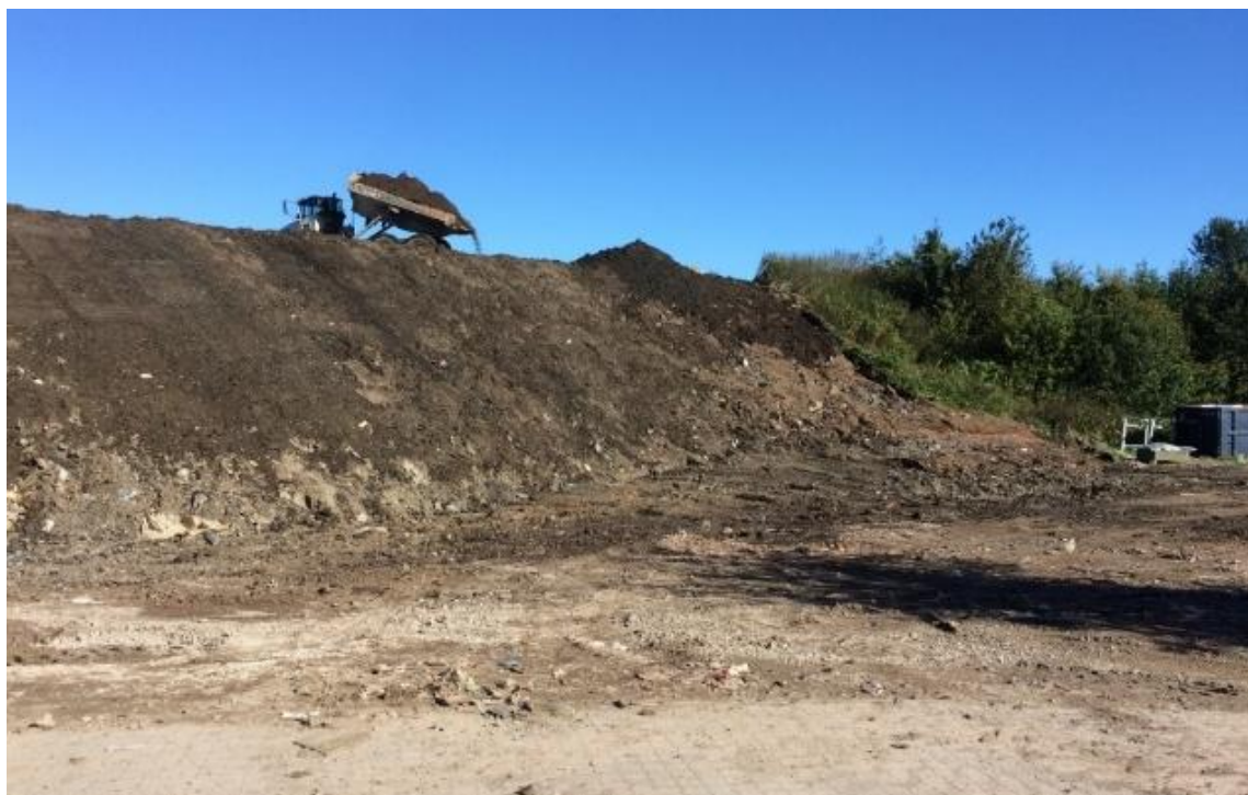
Figure 12-12 Site during the rehabilitation operations.
