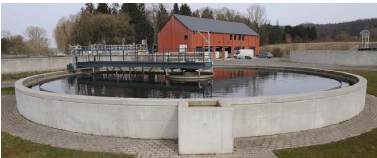
Station d'épuration IBW
